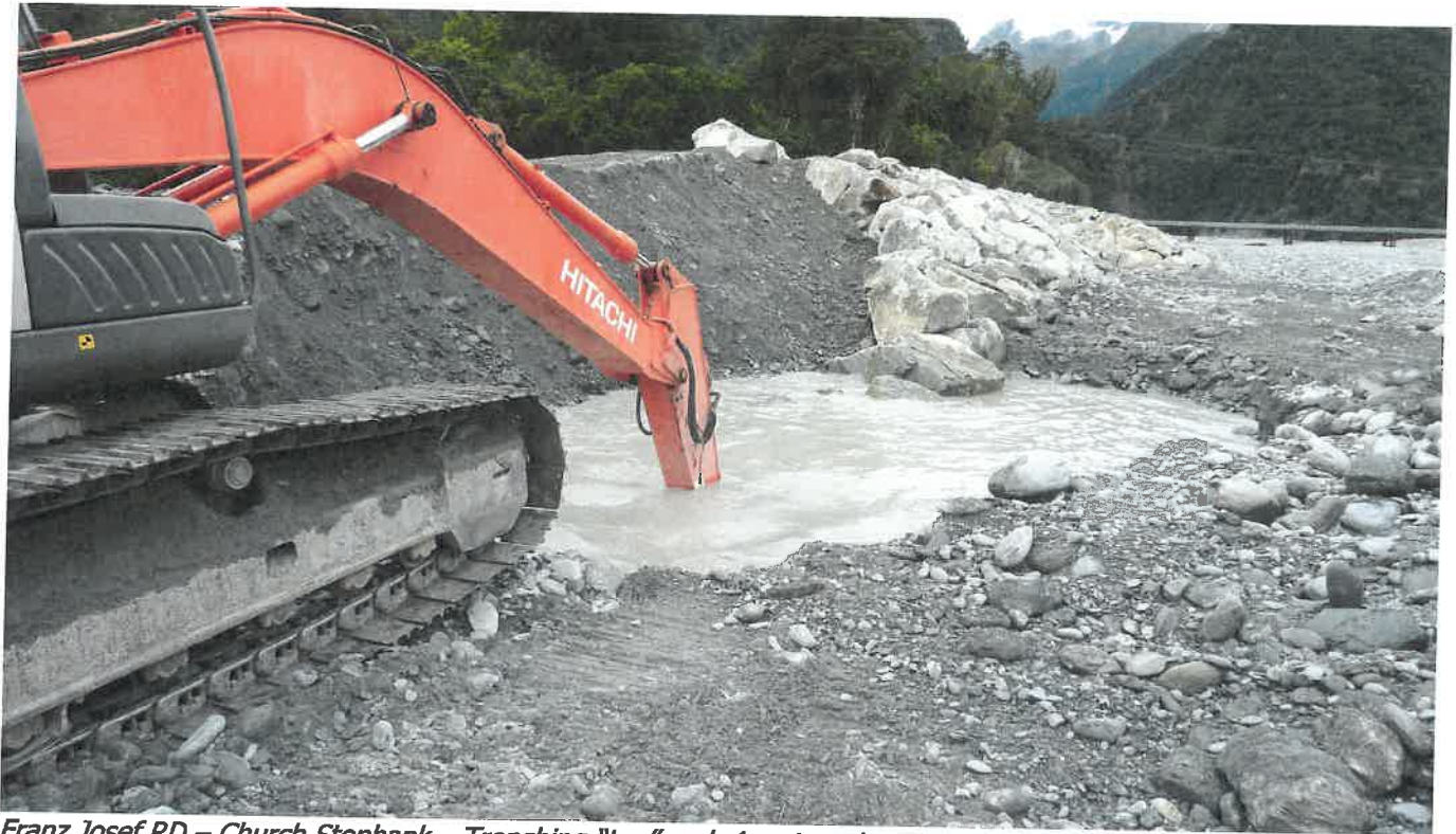
Franz Josef RD – Church Stopbank – Trenching "toe" rock 4 metres deep
