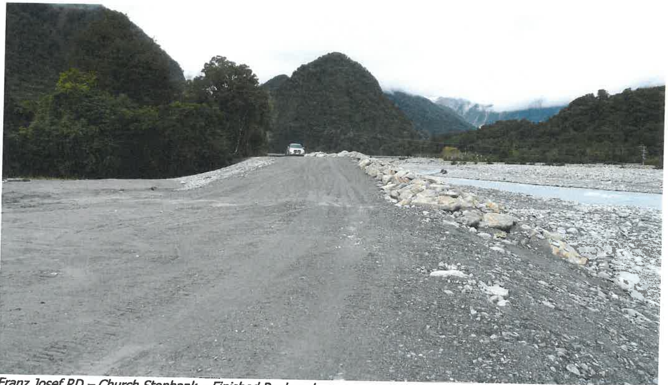
Franz Josef RD – Church Stopbank – Finished Rockwork
