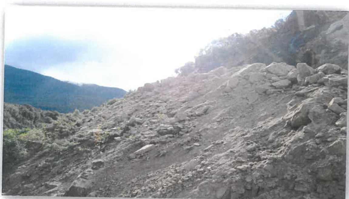
Safety bund below overhang
