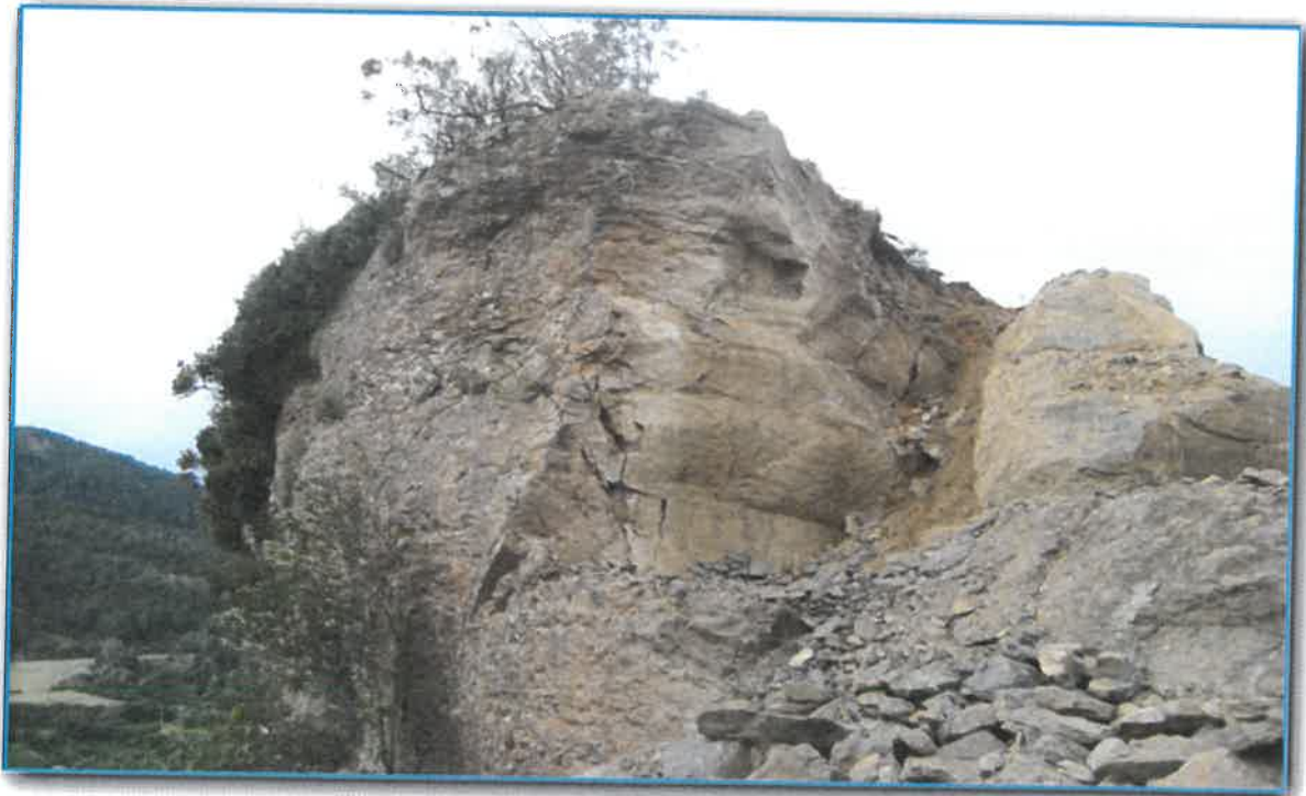
Pinnacle rock after blasting
