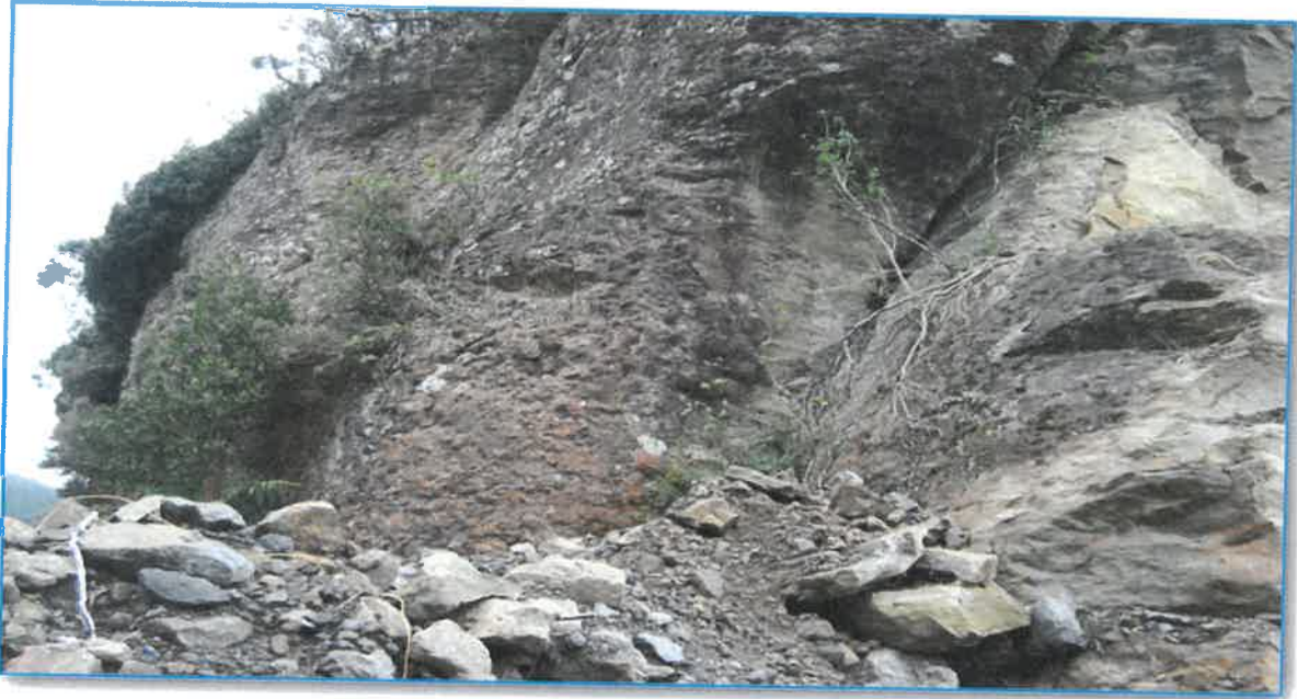
Pinnacle prior to rock removal.
